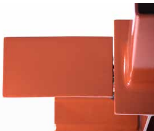
▲ AESS 4: Surfaces filed and sanded.
