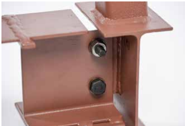
▲ SSS: Bolt head orientation not defined.
