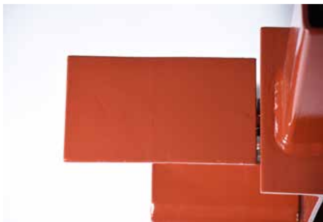
▲ AESS 3: Joint gap tolerances minimized, butt and plug welds ground smooth and filled.
