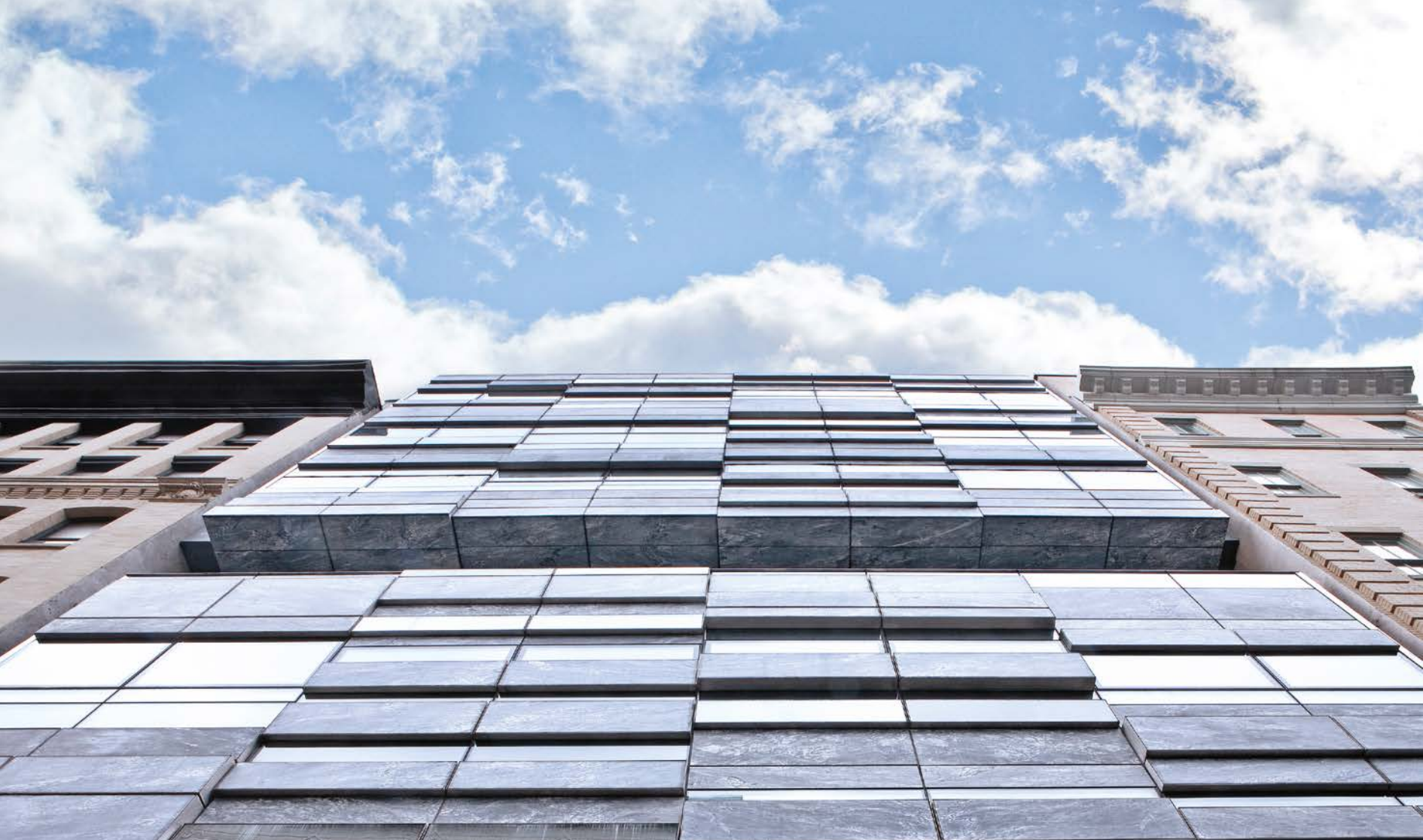
33 Vestry Street New York City, USA Archi-Tectonics
