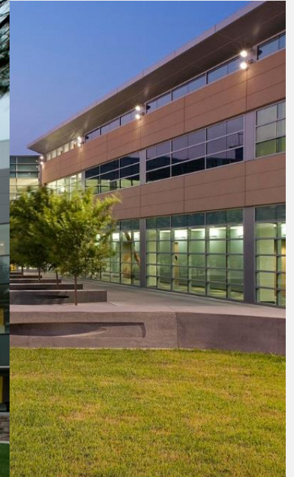
Ohlone Community College Newark Center for Health Sciences and Technology LEED® Platinum
