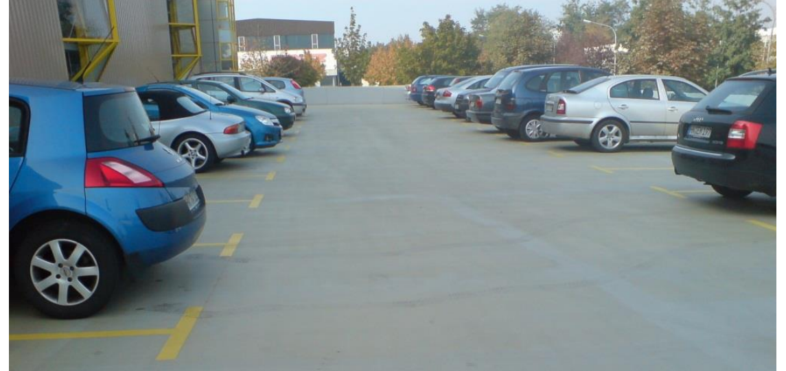
Exposed Carpark Deck
