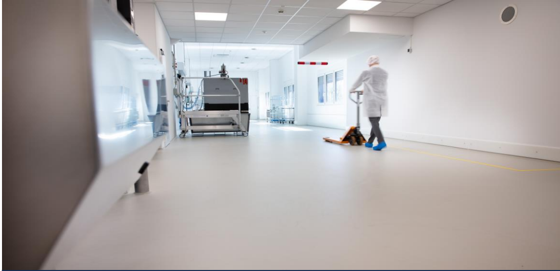
Pharmaceutical Production Plant Walkway
