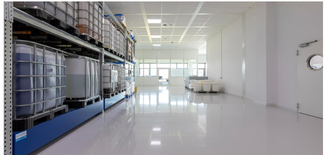
Chemical Storage Facility
