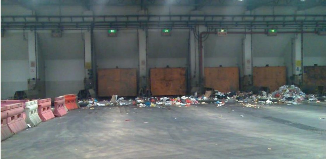
Incineration Plant (Liquid Tight Coating)
